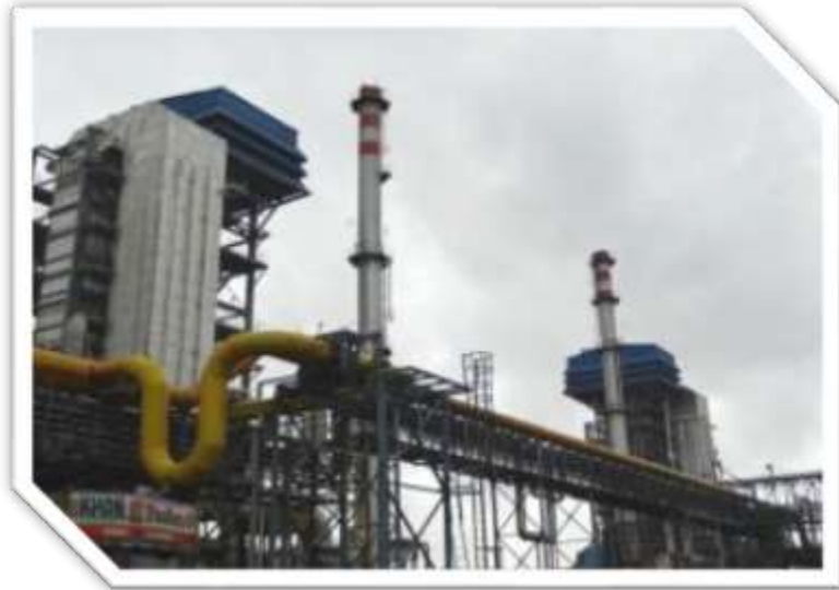
WASTE HEAT RECOVERY POWER PLANT
